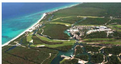
Example of the direct interdependence of maintaining the quality of the natural surroundings and the infrastructure of the Mayakoba tourist complex
